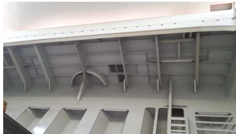
Cross Deck Vulnerable to Sweat
