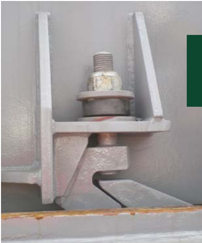
Cleat in Good Condition
