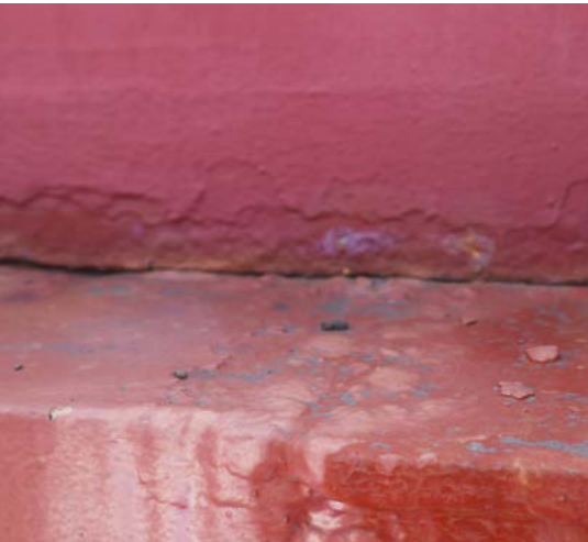
Hatch Cover in Direct Contact with Coaming
