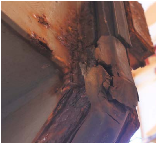
Gasket Cracked
