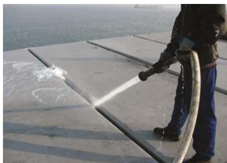
Water Hose Test
