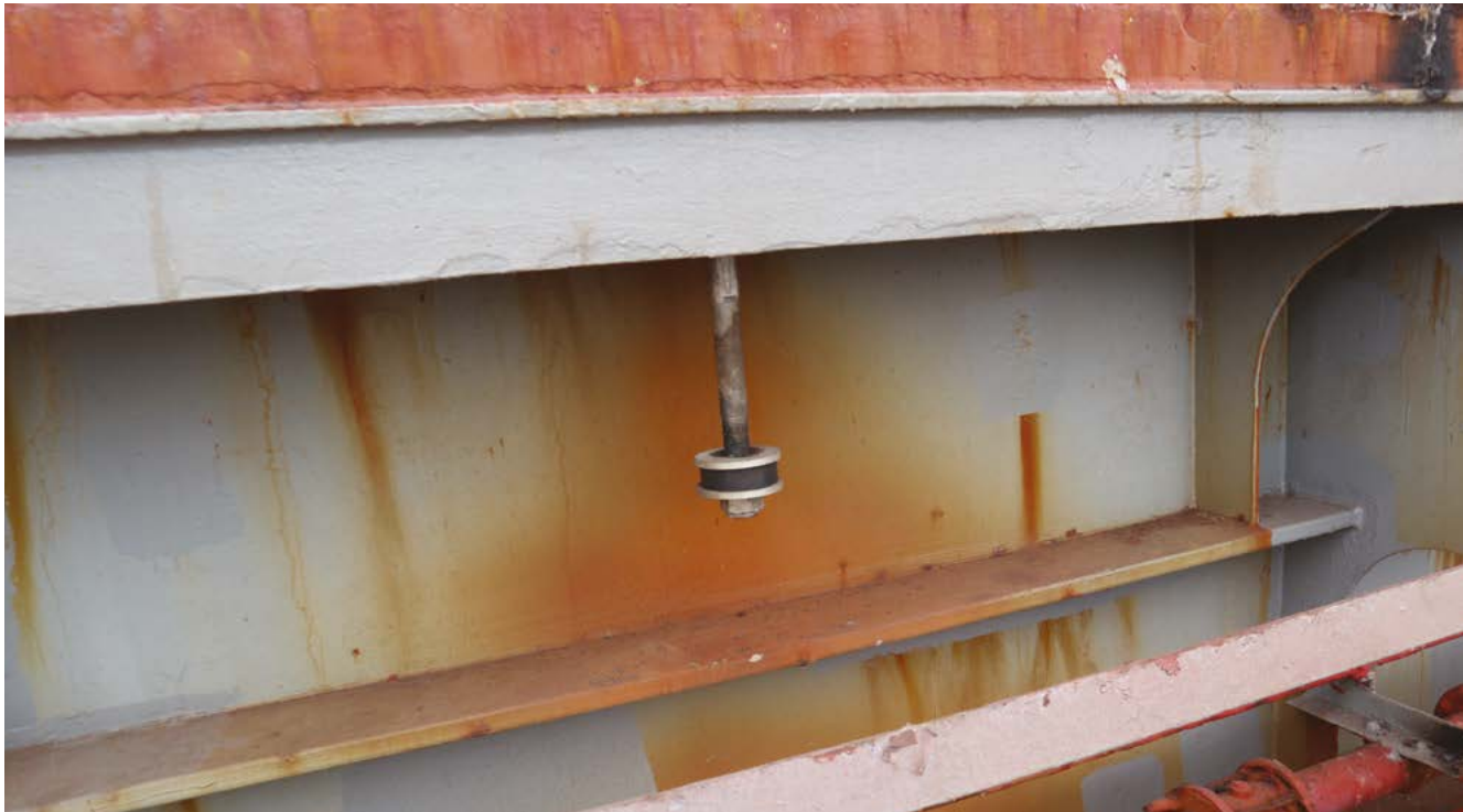
Cleat in Good Condition
