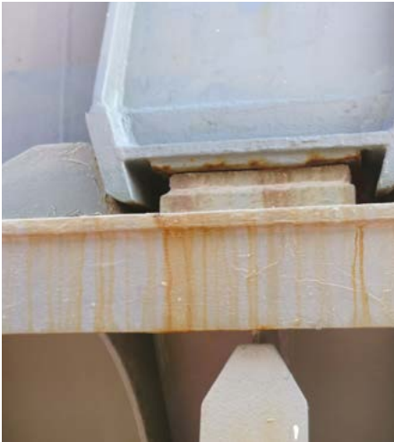
Locators Well Maintained
