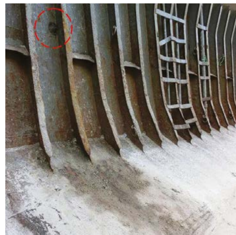
Hull Plate Damaged
